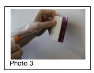
Using smooth even overlapping squeegee strokes to effectively push the air, bubbles, and any wrinkles out of the film as shown in Photos 4 and 5.
